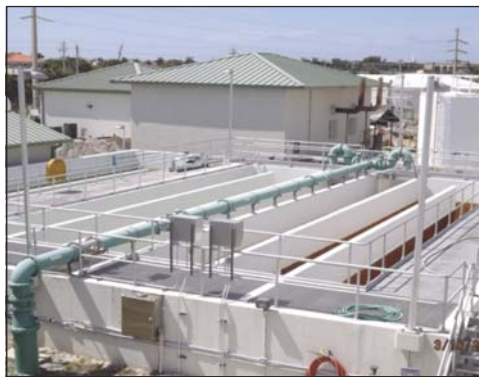
Figure 5. Suspended Solids Meter and Chlorine Contact Chambers
