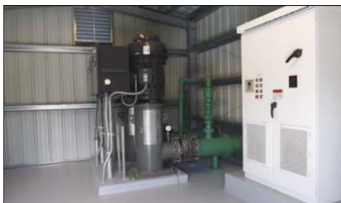
Figure 7. New 400-hp Aquifer Storage and Recovery Feed Pumps
