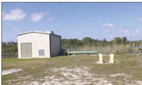
Figure 8. New Aquifer Storage and Recovery Feed Pump Building
