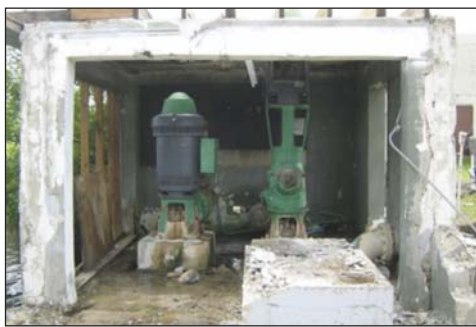
Figure 6. Aquifer Storage and Recovery Pumps During Deconstruction
